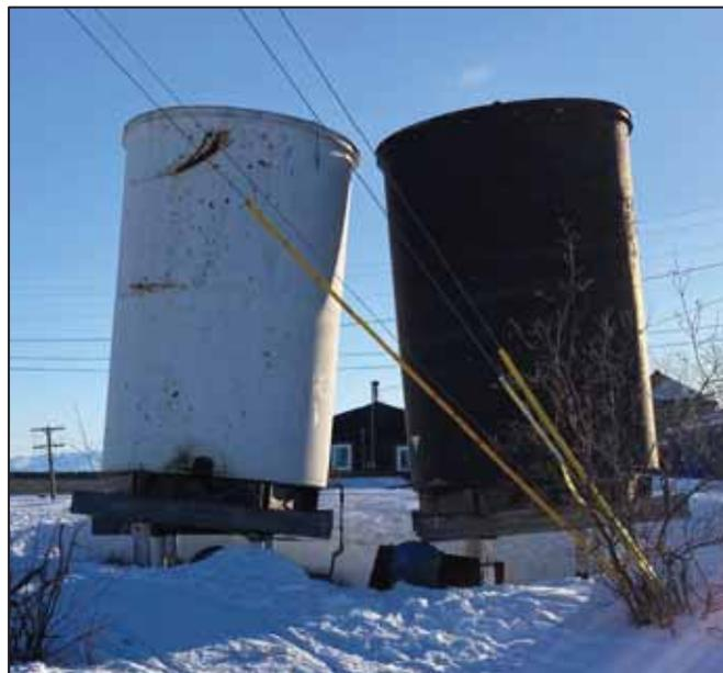
*Figure 13. Aging Fuel Tanks in the Region*
