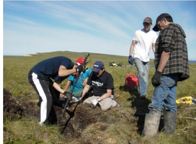
Installing plate anchors; D. Vaught photo
