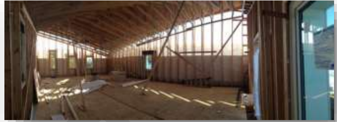
Buckland prototype house under construction.
