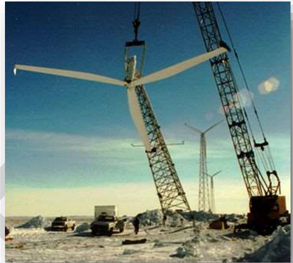
Kotzebue Electric Association wind turbine being raised. Photo courtesy of KEA.
