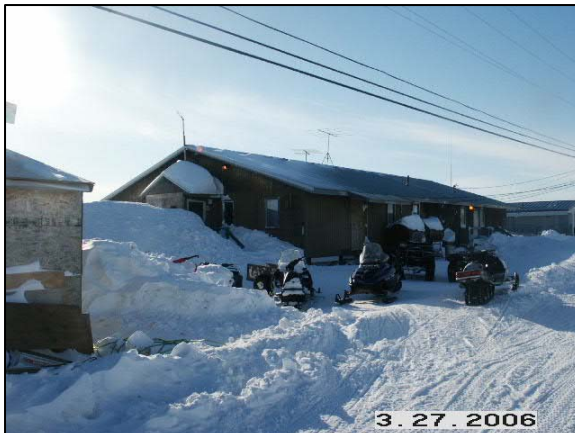
Figure 25: Deering community building with the City and IRA offices, library, holding cell and NANA resource specialist office.
