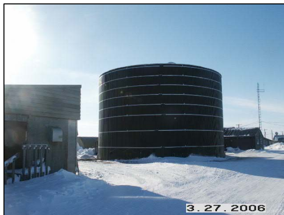
Figure 13: Deering water storage tank.
