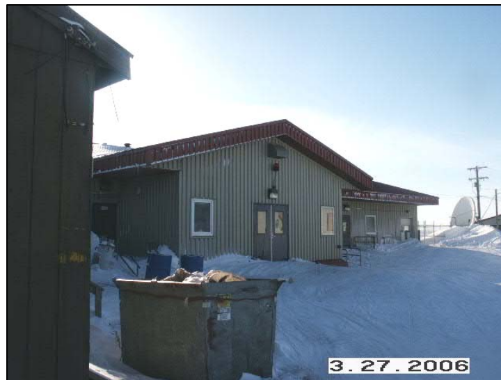
Figure 17: Ipnatchiaq Electric power house and City washeteria building with community trash bin in front.
