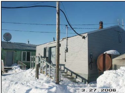
Figure 20: OTZ building in Deering.
