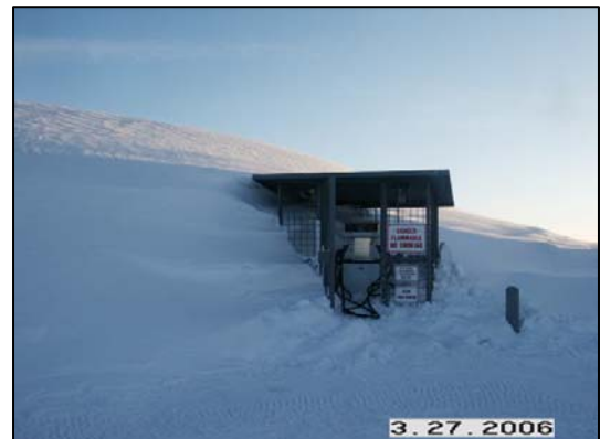
Figure 9: Native Village of Deering fuel/gas pump.
