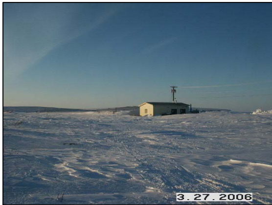
Figure 15: sewer system building by the Deering sewage lagoon.
