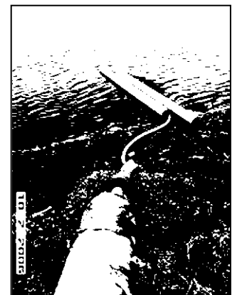
Figure 17: water intake equipment at the Buckland River.
